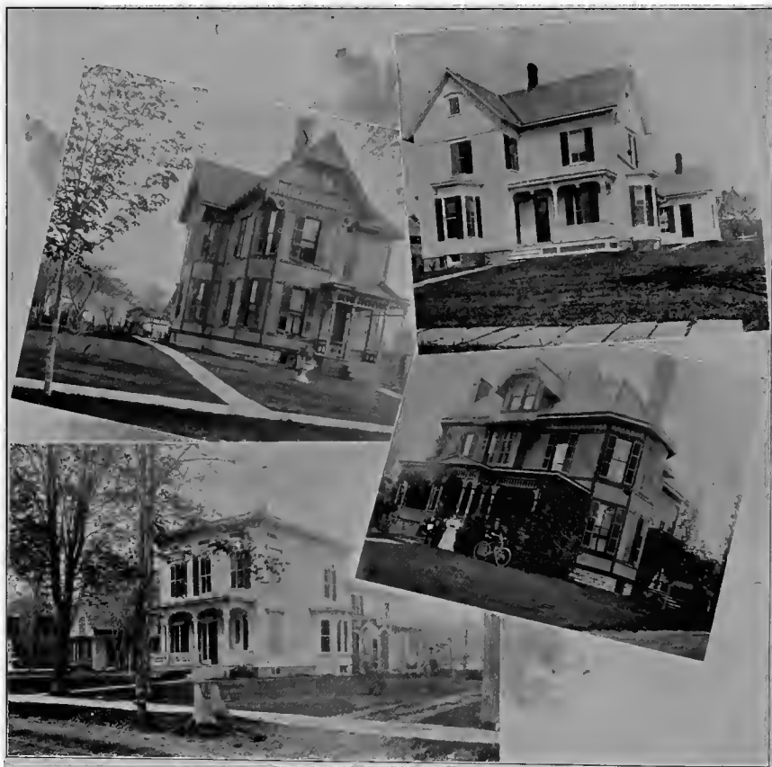
T. E. DORNET'S RESIDENCE, W. MAIN ST. J. H. CRANDALL'S RESIDENCE, GRAND ST.
